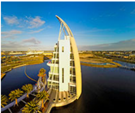
Exploration Tower at Port Canaveral
